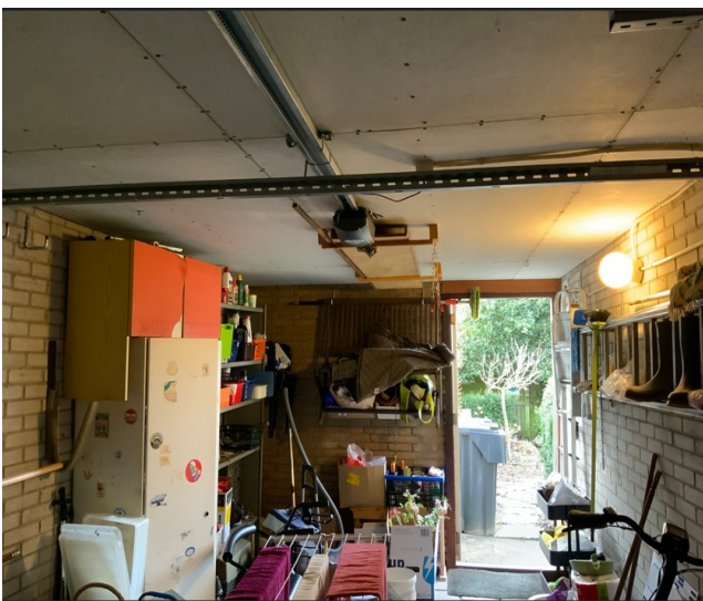
Plafond in Garage
